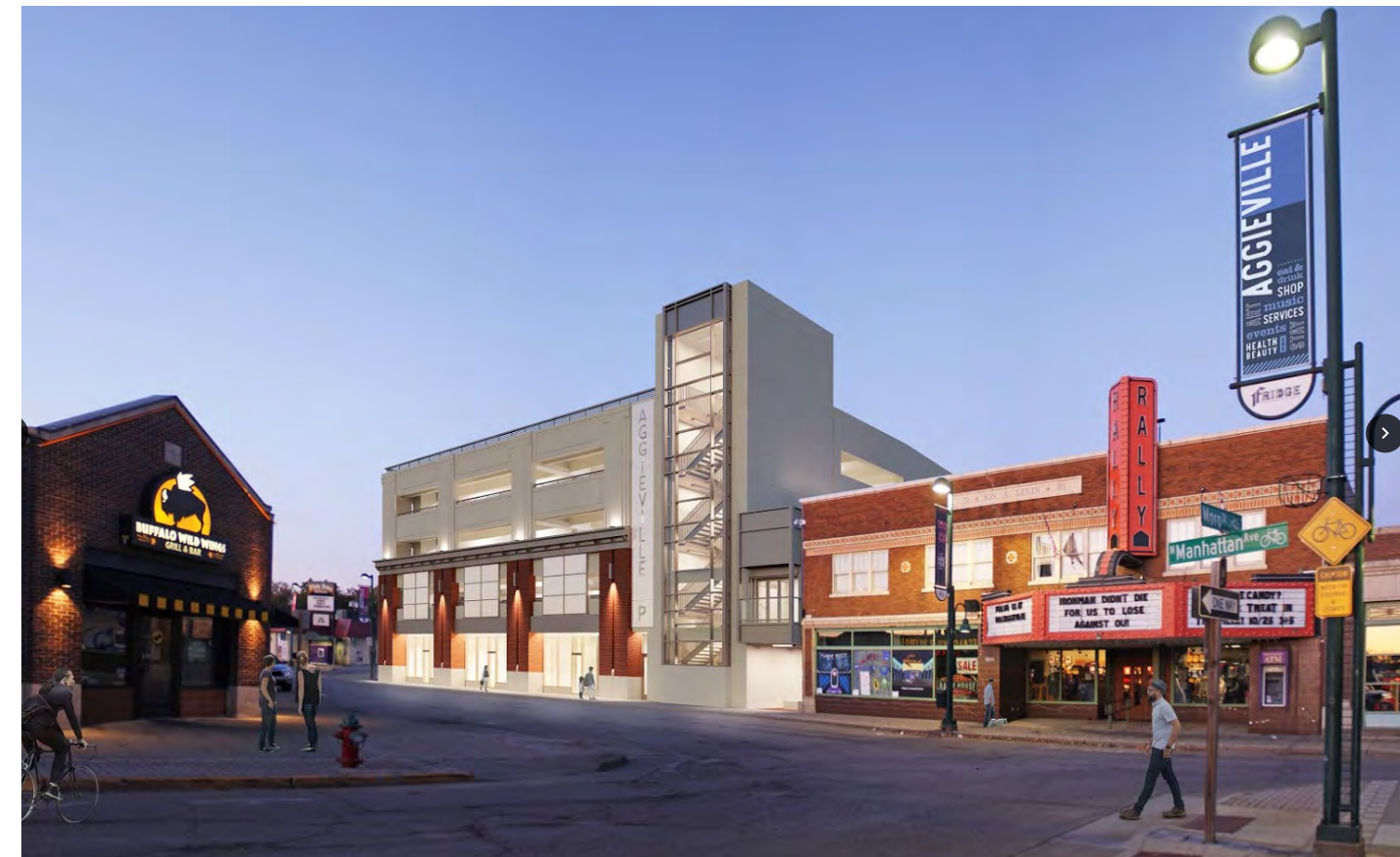
Construction of the Aggieville parking garage broke ground on December 11, 2020
